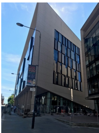
Figure 1. The Technology & Innovation Centre, University of Strathclyde, Glasgow, UK.
